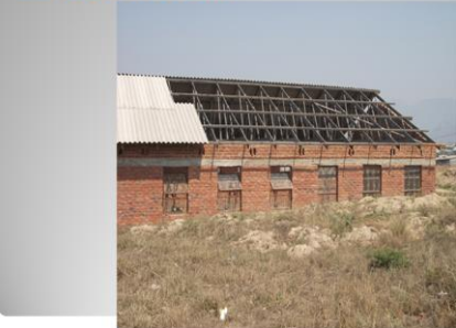
One of the blocks under construction
